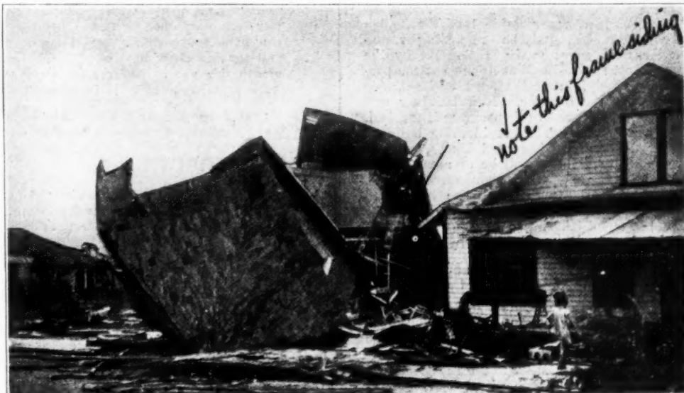
"This is a fair sample of what happened to concrete block walls," writes W. F. Shaw, to whom we are indebted for this and other photographs from the storm area. Note the wood shingle roof from the wrecked building.
